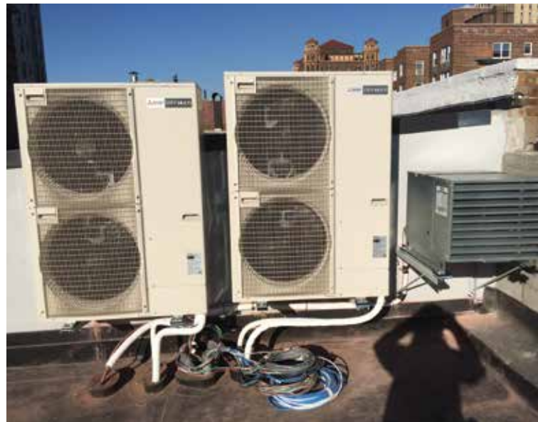
Two 4-ton Mitsubishi VRF condensing units heat and cool this 7,500 sq ft Brooklyn Heights Passive House. A conventionally built home this size would need at least twice the amount of cooling and heating.
