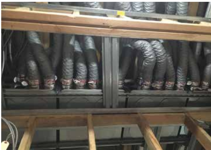
New UL-Approved Zehnder ComfoFlex 3" diameter supply and extract air ducts. These ducts course above the ceilings and behind the walls of passive homes to ventilation registers.
