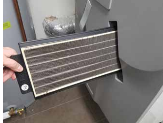
Fresh outdoor air intake around the clock can quickly clog up air filters. ERV filters must be changed regularly to ensure proper ventilation of passive homes.
